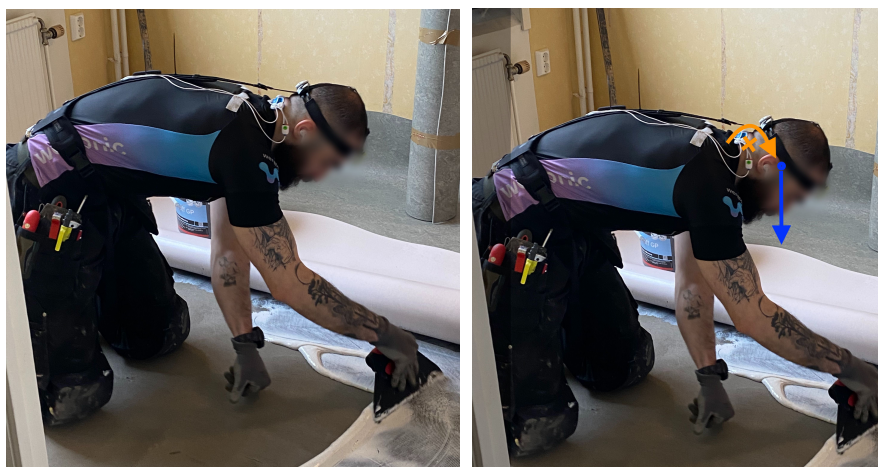
Figure A1 A photograph of a typical work posture and the basis for the biomechanical calculation (right) with the torque equilibrium at the neck (orange) and the gravitational force of the head (blue).
